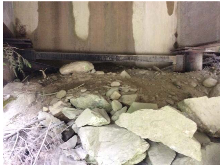
Left Bank Abutment when facing downstream
