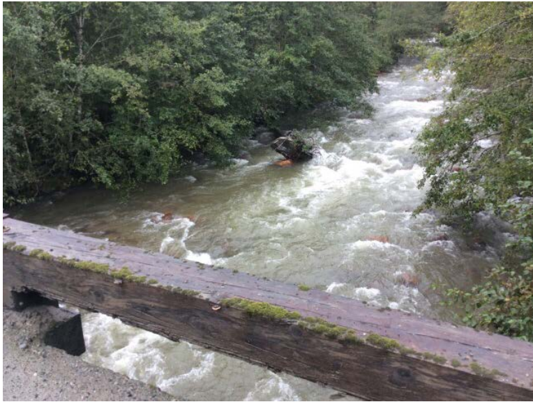
Upstream from Crossing
