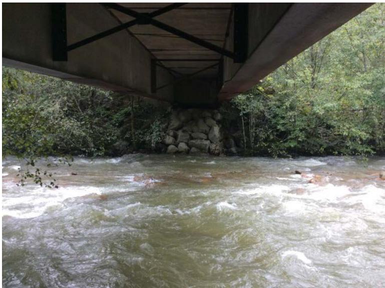
Right Bank Abutment when facing downstream
